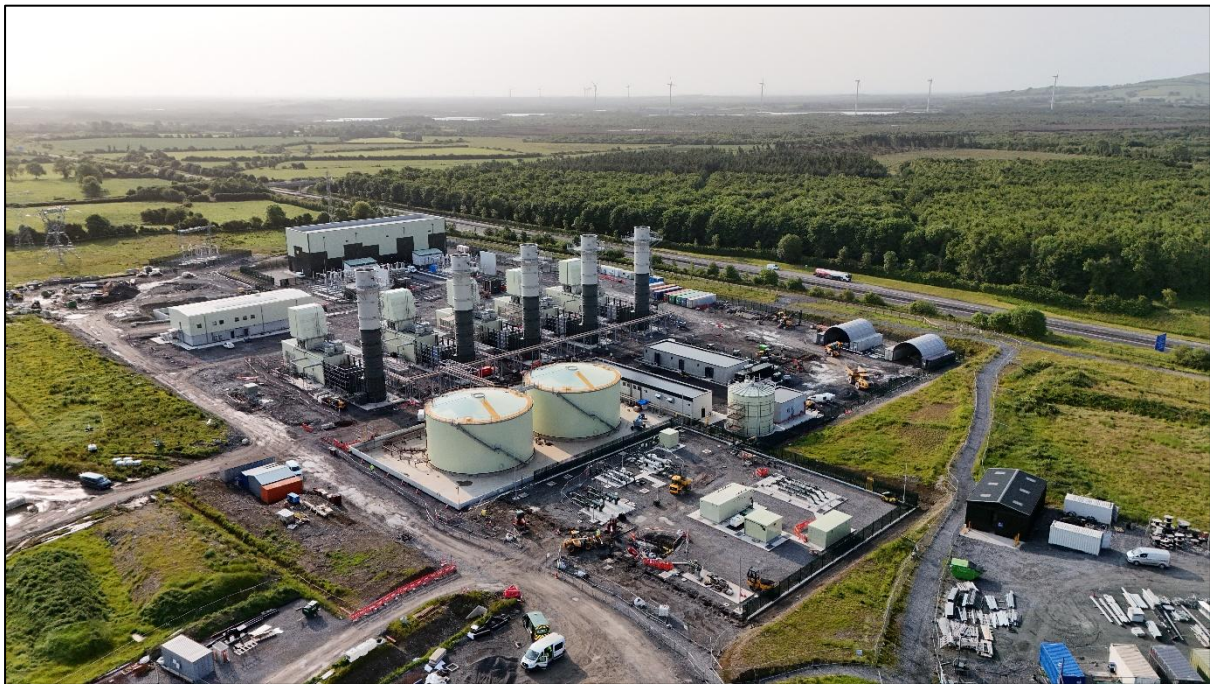
Figure 2.1 Aerial View of the Castlelost Flexgen and GIS Substation (June 2025)
