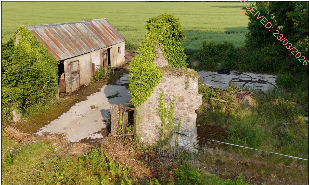
Figure 2.6 Photograph shed and derelict structure to be demolished
